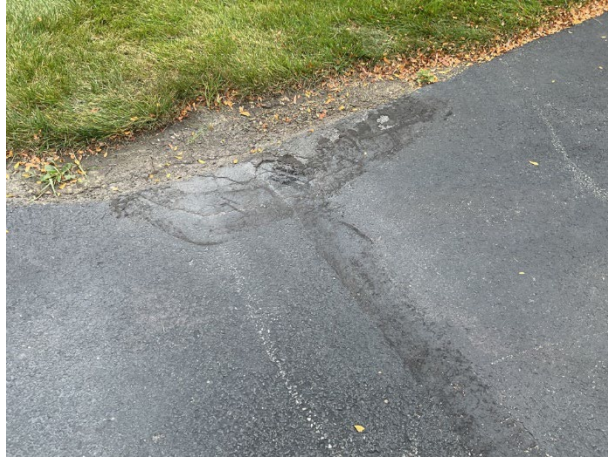
Pavement cracks and previous repairs
