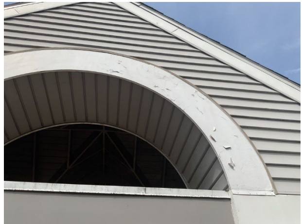
Paint finish deterioration
